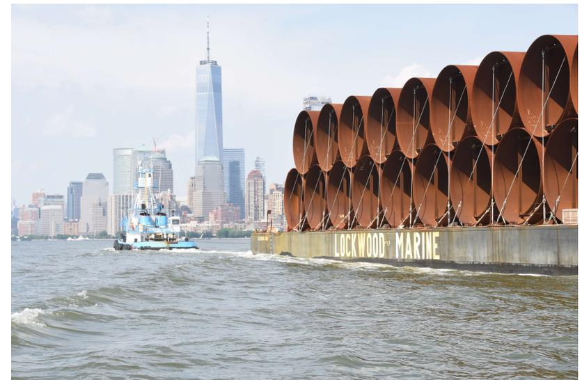
Steel liners for the Delaware Aqueduct Bypass Tunnel with Freedom Tower in background
