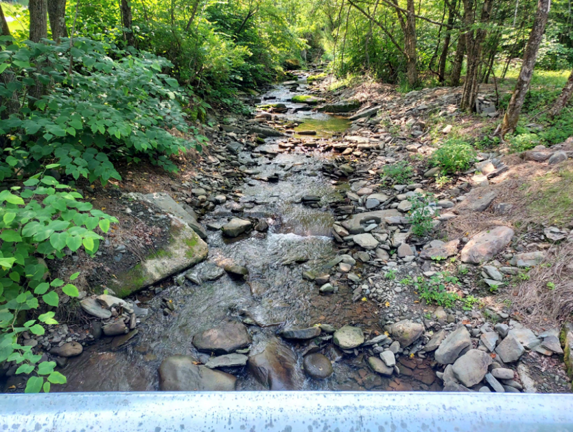
Cooks Brook facing upstream, 9 months post project: grade controls
