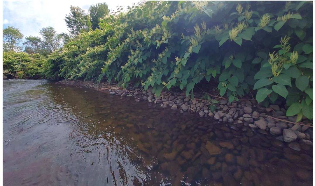
Erosion beneath knotweed on upstream bank
