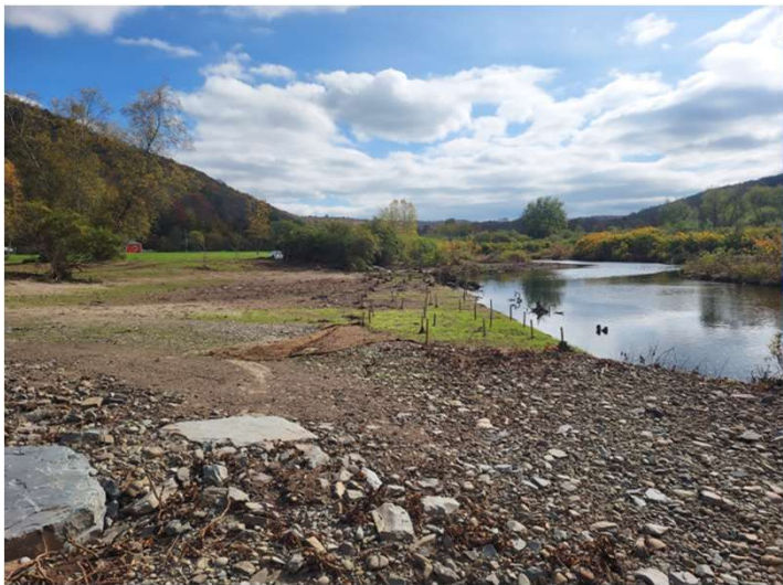
Realigned bank; improved floodplain access, toe wood for protection and habitat.
